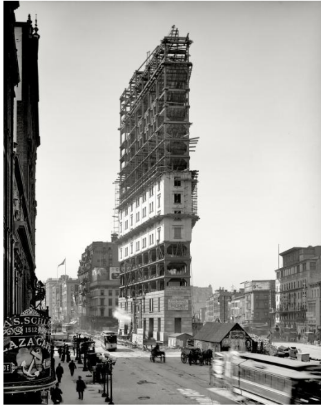
Figure 11. Times Square One under construction (Source: Wikipedia Commons)
